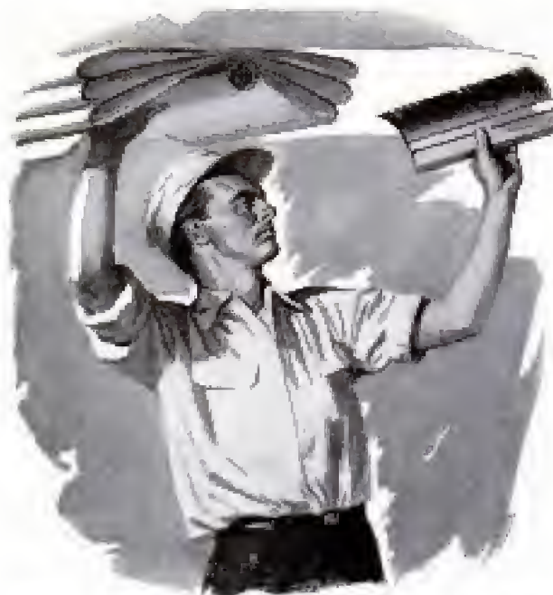
When papering ceiling, the paper is carried loosely folded back and forth across a stick or odd roll of paper. It unfolds easily as you cross the room
